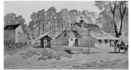
Howard's Tavern as it appeared in 1776; it was demolished in 1880. The tavern was located near the present-day intersection of Fulton Street and Jamaica Avenue.
